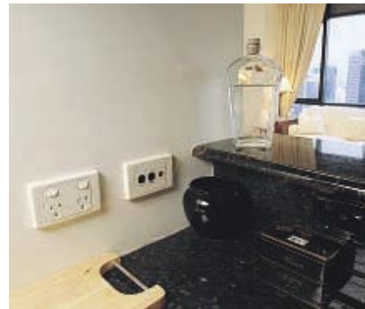
Functions can be reprogrammed at the computer interface point, situated above the kitchen bench.
