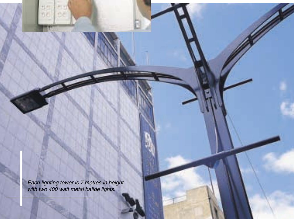
One of two PE Sensors that automatically operate all 21 towers at sunset.
