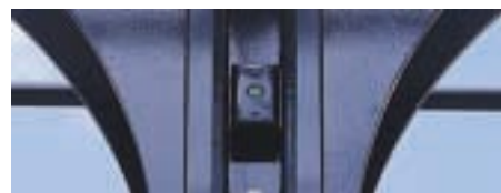
One of two PE Sensors that automatically operate all 21 towers at sunset.
