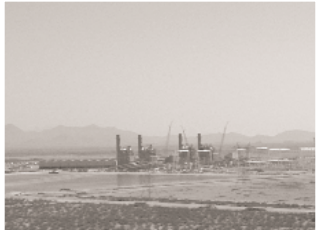
Salt River Project's Hassayampa Switchyard
